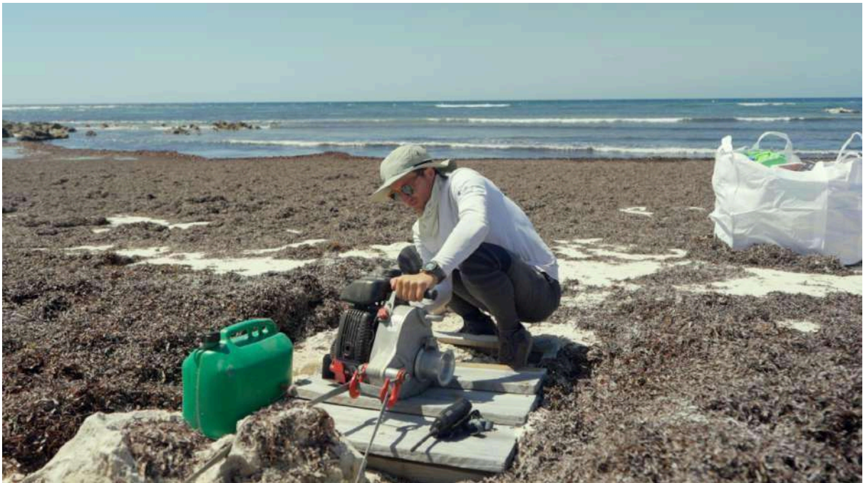
Installation of the forestry winch to tow the platform ashore
