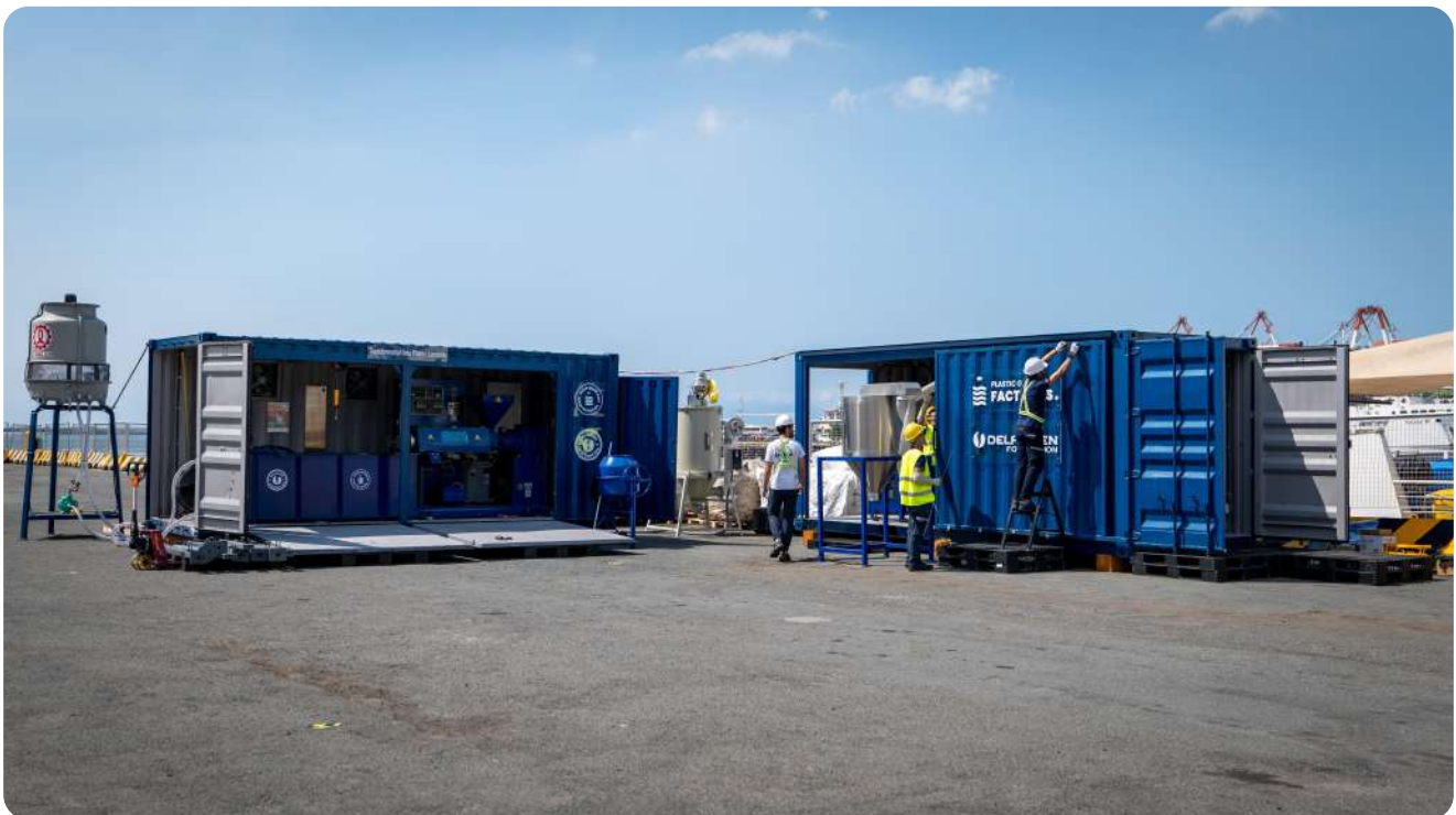
FIG-04 Unloading a containerized POF unit at the dock of Manila, Philippines.
