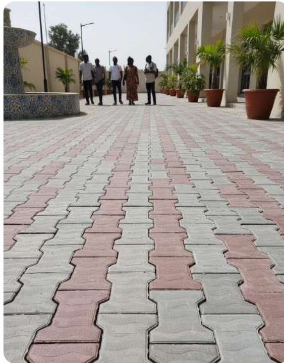
FIG-03 Recycled plastic pavers, close-up.
